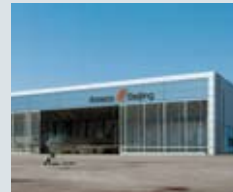
Ameco A380 Hangar, Beijing, China
